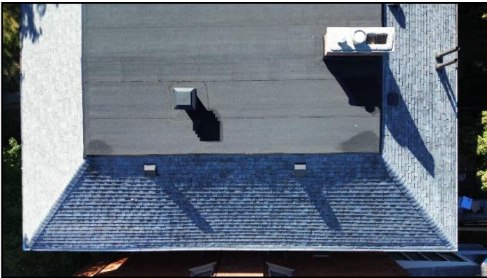
2. Full roof view
