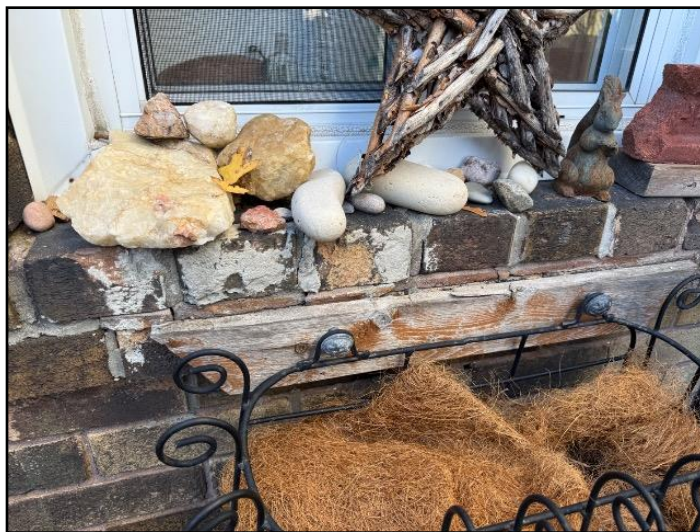
20. Sill deteriorated
