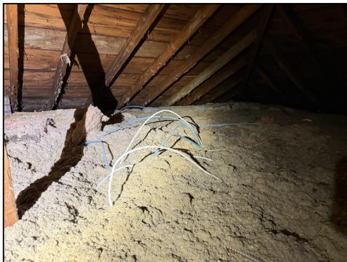
25. Exposed in attics
