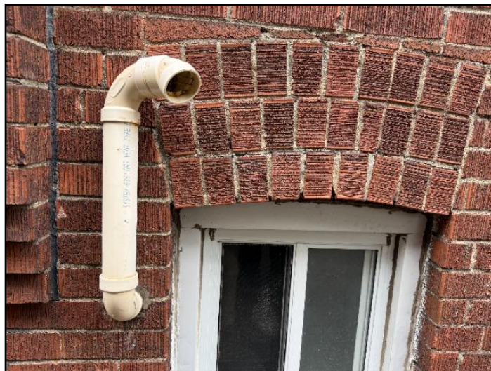
19. Vent termination clearance concern
