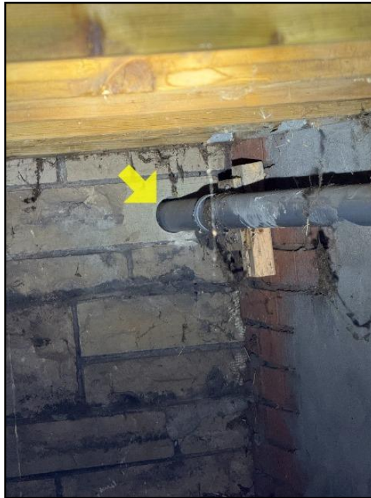
4. one example where conduit enters wall
