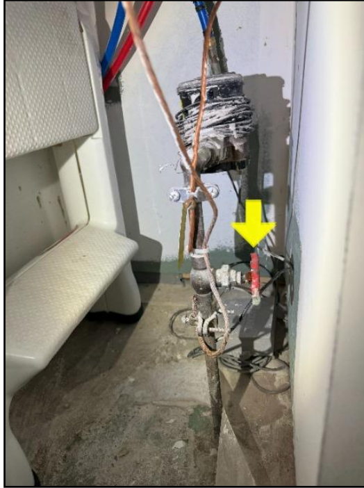
18. Main water shut off valve - Basement
