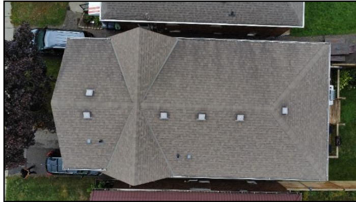
1. Asphalt shingles
