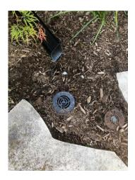
There is a drywell (via a drain) below the front lawn to disperse water that discharges from the front downspout.
